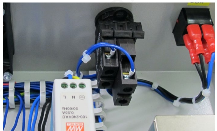
Fig. 4: Assembly of button, LED element, contact element
