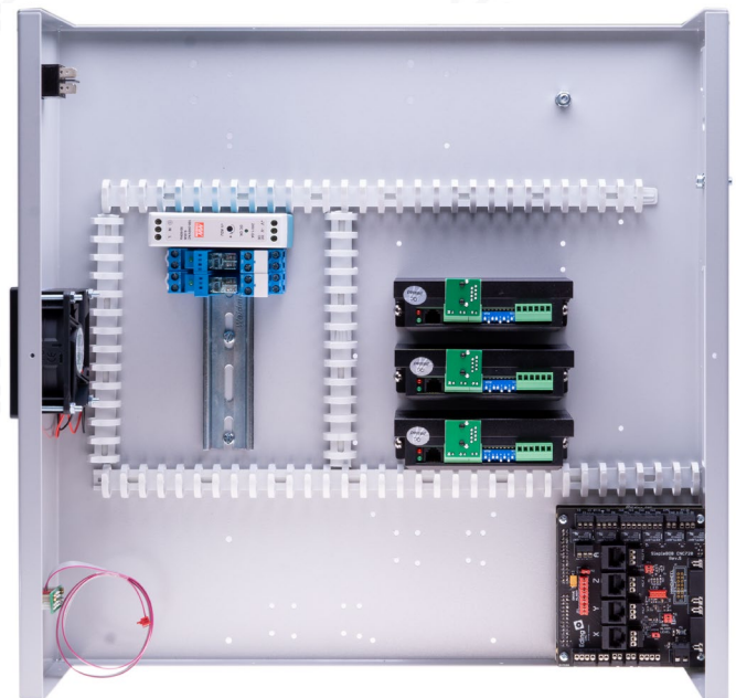
Fig. 13: Housing with internals before the start of the wiring
